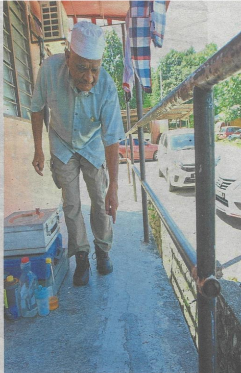
Mohammad Saidin showing cracks that he claims to have reappeared on the floor after the repair work. — Photos: LOW LAY PHON/The Star
