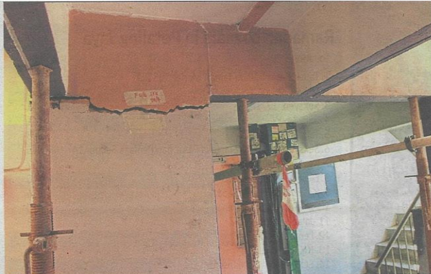
Cracks are seen on walls and iron beams have been placed near the staircase (right) to support the structure.
